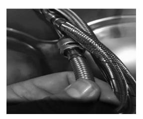
**Step three** – Attach Hot (red) and Cold (blue) supply lines hand thread the supply line and gently tighted with a wrench.
